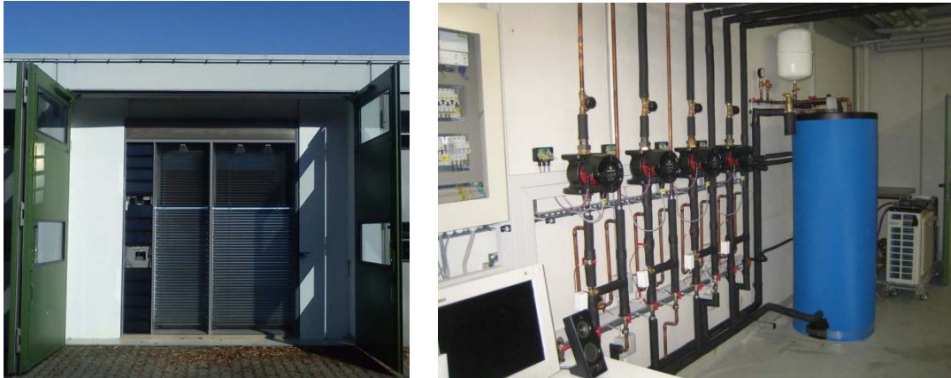
Figure 2.3: Test façade with test room and hydraulic systems
