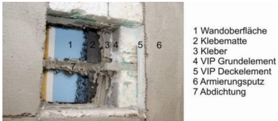
Figure 4: Innendämmaufbau_VIP.jpg Component opening with layer indication of the interior insulation at the east wall.
