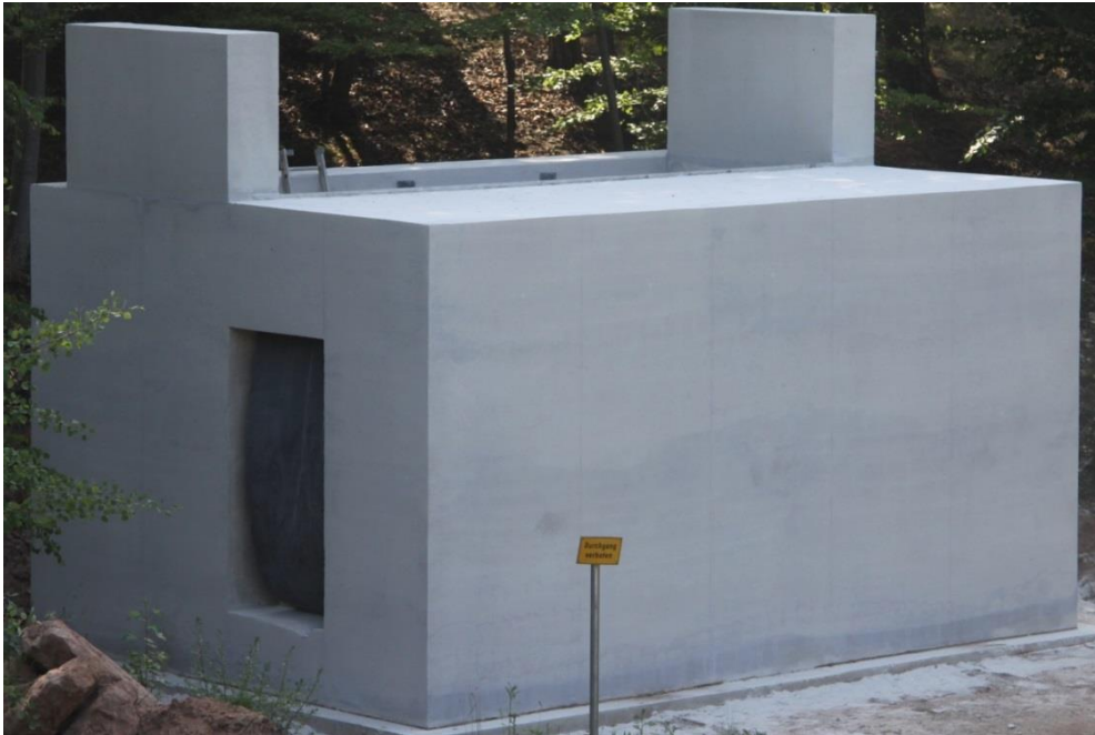
Figure 4: Experimental building made of architectural lightweight concrete, after concrete work
