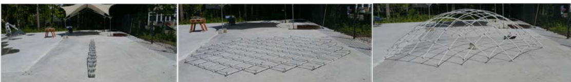
Image 1.6: Sequence of the erection process for the mock-up
