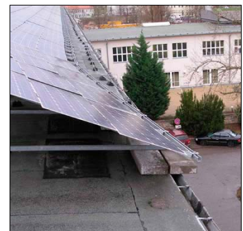
A 6: Horizontal movement of solar facilities over the unsecured roof edge
