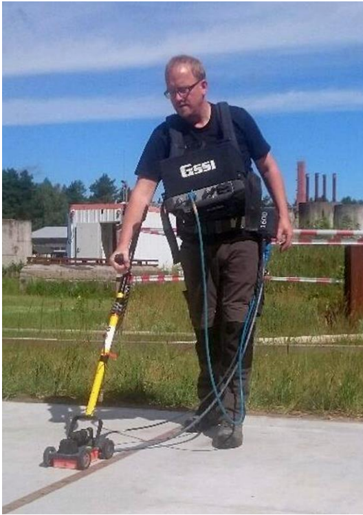
Figure 3: Radar measurements by Implenia Construction AG on top of the REFUND test slab (BAM-TTS, Horstwalde) to determine rebar position and slab thickness. File: Figure3.jpg
