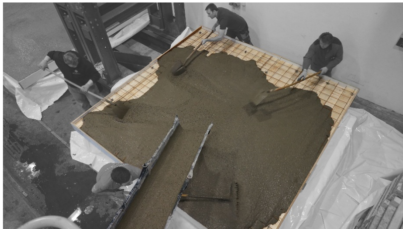
Figure 5: Building the concrete layer
