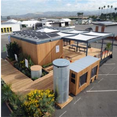
Fig. 1 Exterior view of nexushaus (south-west view)
