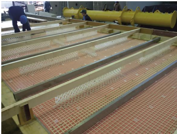
Fig. 3: reinforcement of the first facing with shear connectors secured against floating
