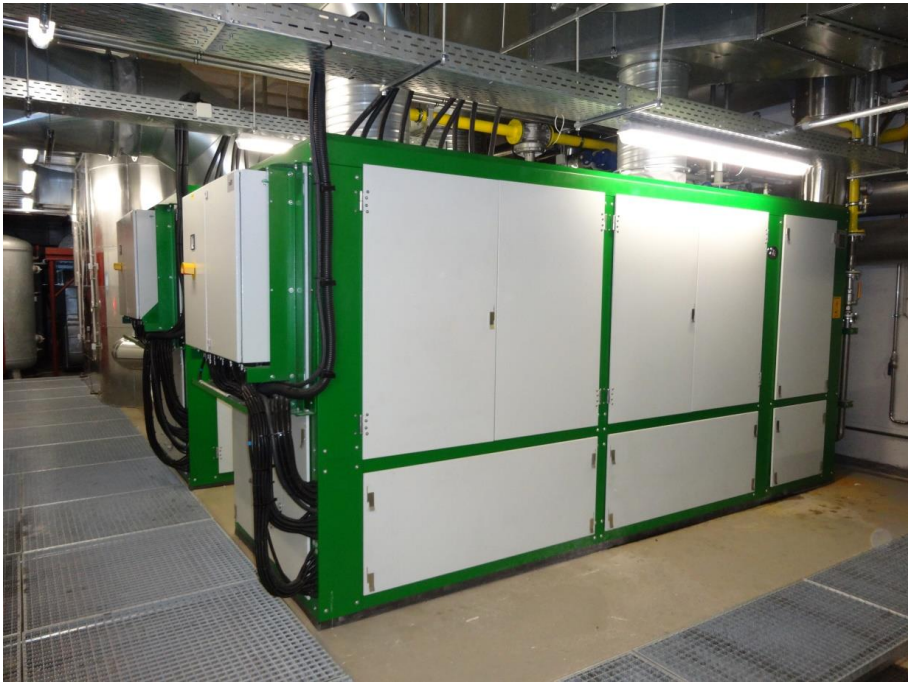
Fig. 4: CHP-units of CHP-plant D
