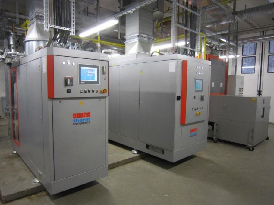
Fig. 2: CHP-units of CHP-plant A
