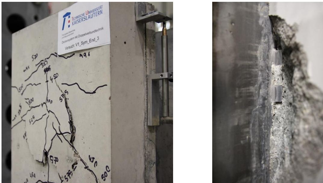
Figure 4: Concrete cone failure on the outside (left) and on the inside (right) of the experiment V1-Sym-End-3
