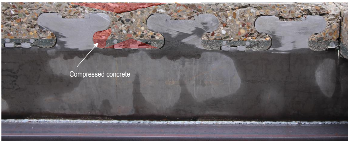
Figure 7: Cut-out of the saw cut along the shear joint of "final state" specimen
