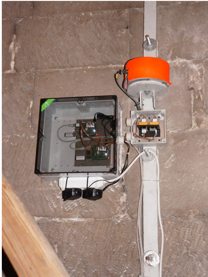
Figure 4: Installed measurement system inside a church tower.
