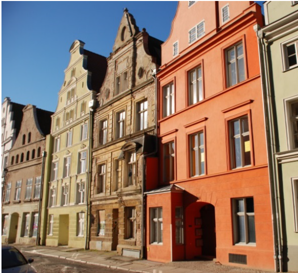
Fig. 2 - Decorated gabled houses in Mönchstraße in Stralsund (some with façade damages), A1
