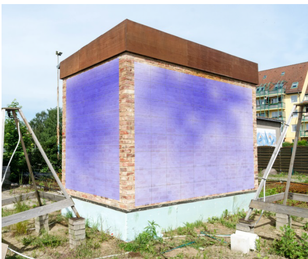
Fig. 7 - Moisture distribution on south and east façades of the artificial irrigated test building 5, A2
