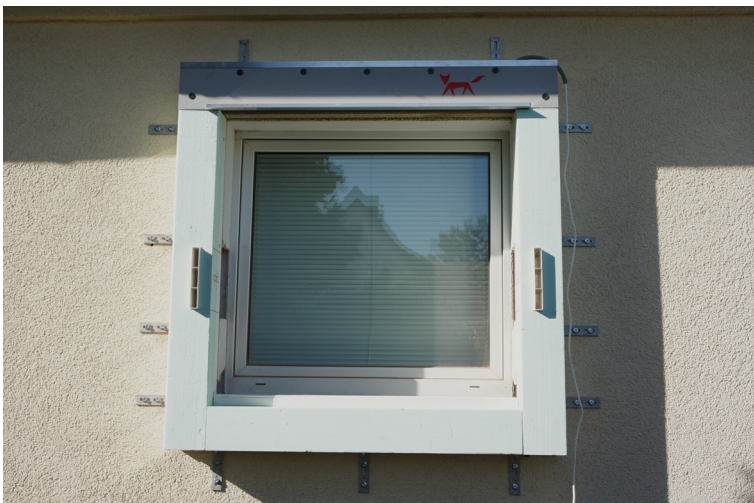
Fig 4: Fixing the window machine without external thermal insulation system.jpg
