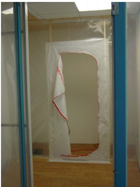
Figure 2: View through the anteroom of the setup at a prefabricated partition with zip.
