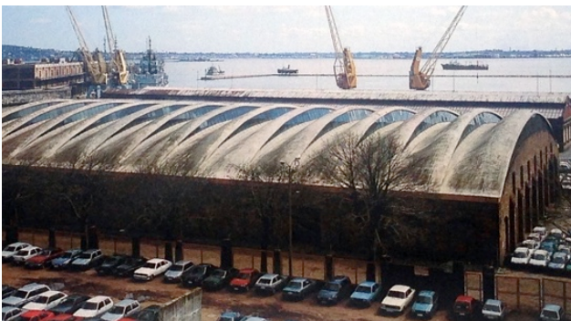
Figure 1: External view - Depositas Montevideo, A1
