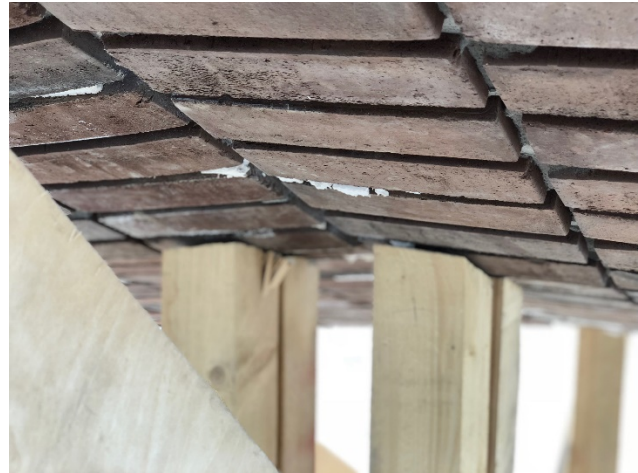
Figure 9: Test series 2: Falsework - support for precast element, A2
