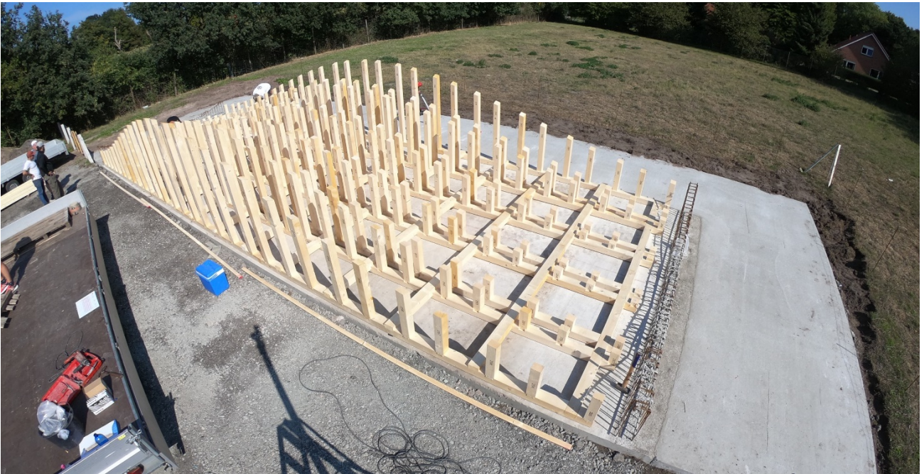
Figure 11: Assembled falsework without transverse bracing, A2
