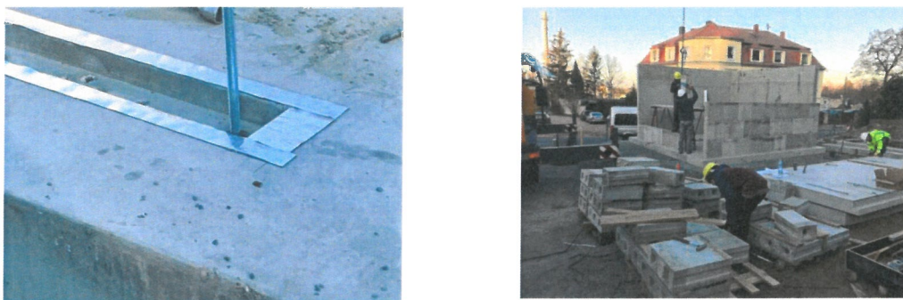
Figure 16 Reassembly at the new location. Sealing against rising moisture on the concrete slab (left) – wall assembly (right)
