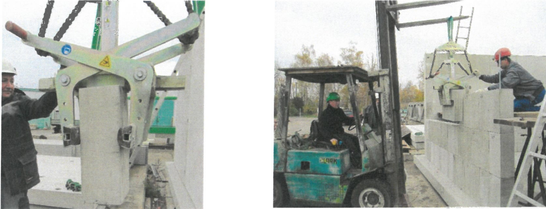
Figure 15 Dismantling of a RC concrete stone with the angled pincers
