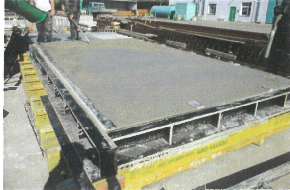
Figure 13 RC-ceiling slab 1, concreting
