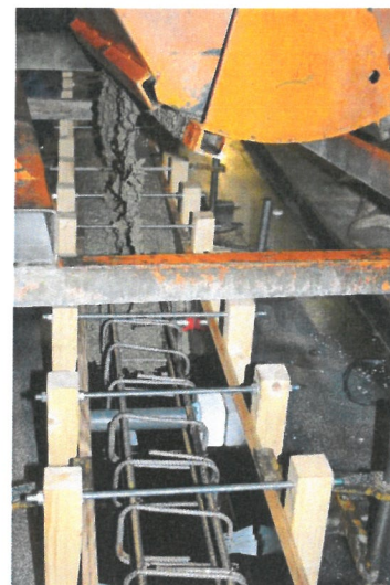
Figure 11 RC-beam, filling the RC beam
