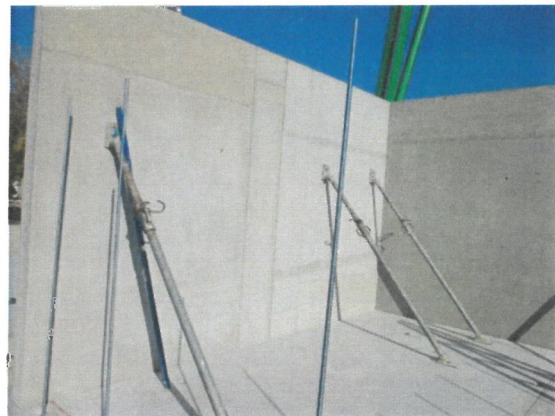
Figure 14 Assembly of the wall slabs by means of assembly supports
