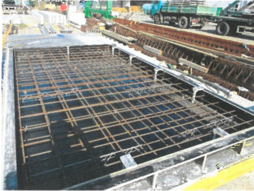
Figure 12 RC ceiling slab 1, formwork, connection technique
