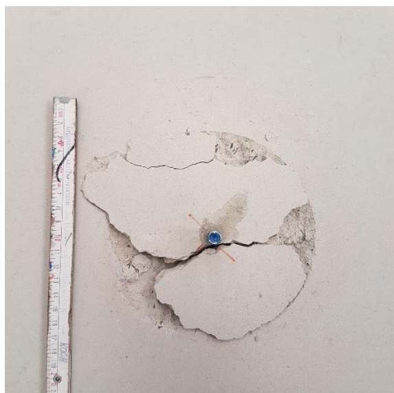
Abbildung 8-83 Bau KS M10x50mm Test 3
