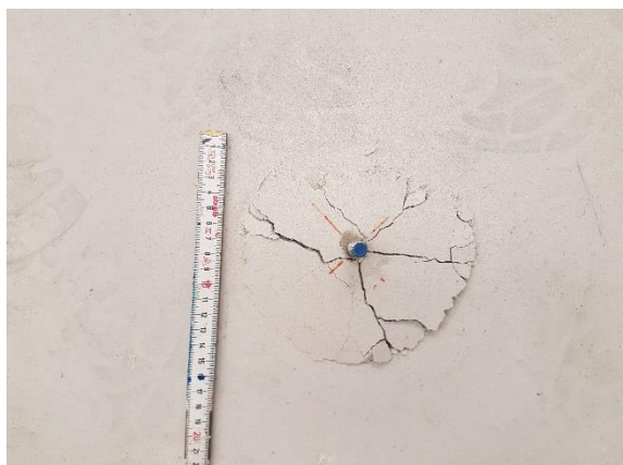
Abbildung 8-82 Bau KS M10x50mm Test 2
