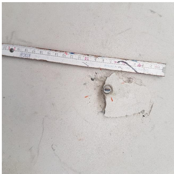
Abbildung 8-81 Bau KS M10x50mm Test 1
